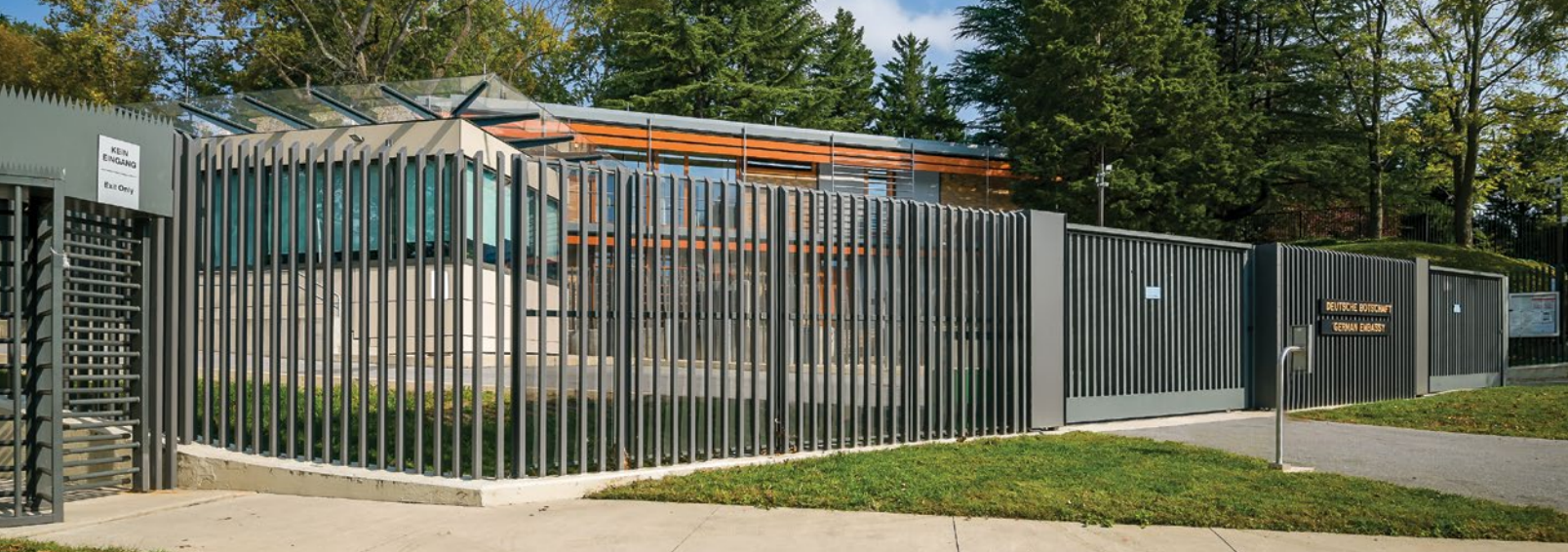
Hercules fencing outside the German Embassy at 4645 Reservoir Rd NW. Photos courtesy of Hercules.
